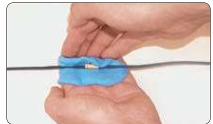
Insulation of multiple connections
