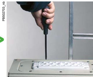
Make a Small Hole in the Membrane
