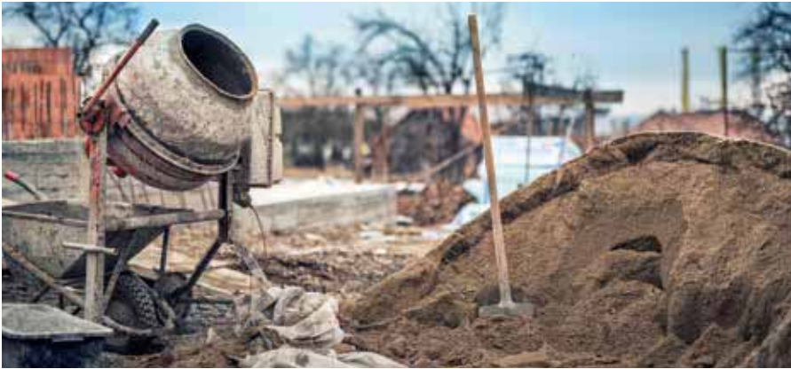
Building construction site
