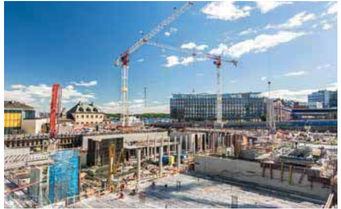
Building construction site
