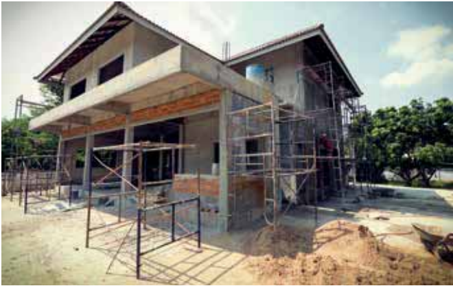
Building construction site
