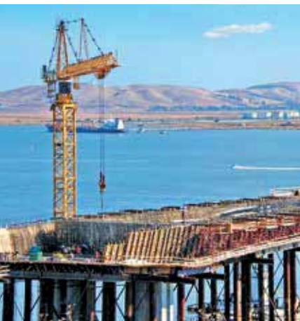
Building construction site
