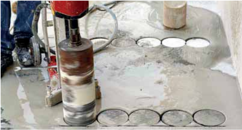
Building construction site
