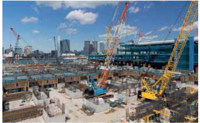
Building construction site
