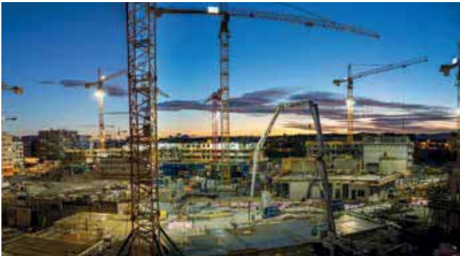
Building construction site
