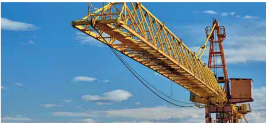
Building construction site
