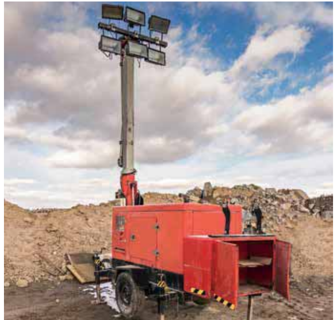
Building construction site
