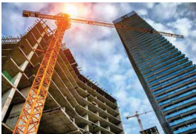
Building construction site
