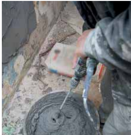
Building construction site
