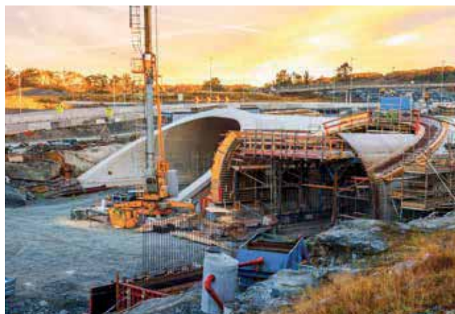
Building construction site
